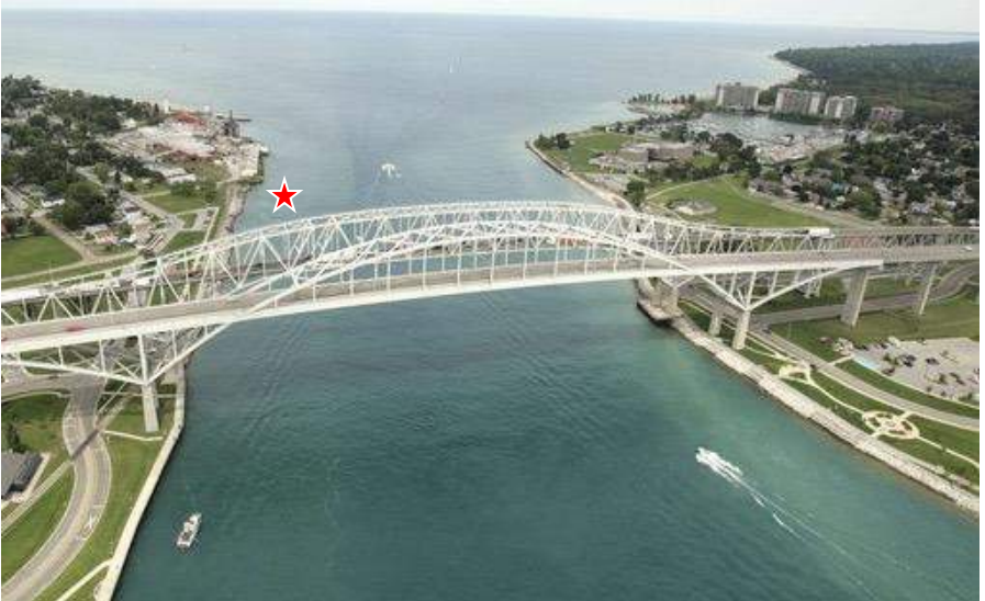
The St. Clair River, Blue Water Bridge.
